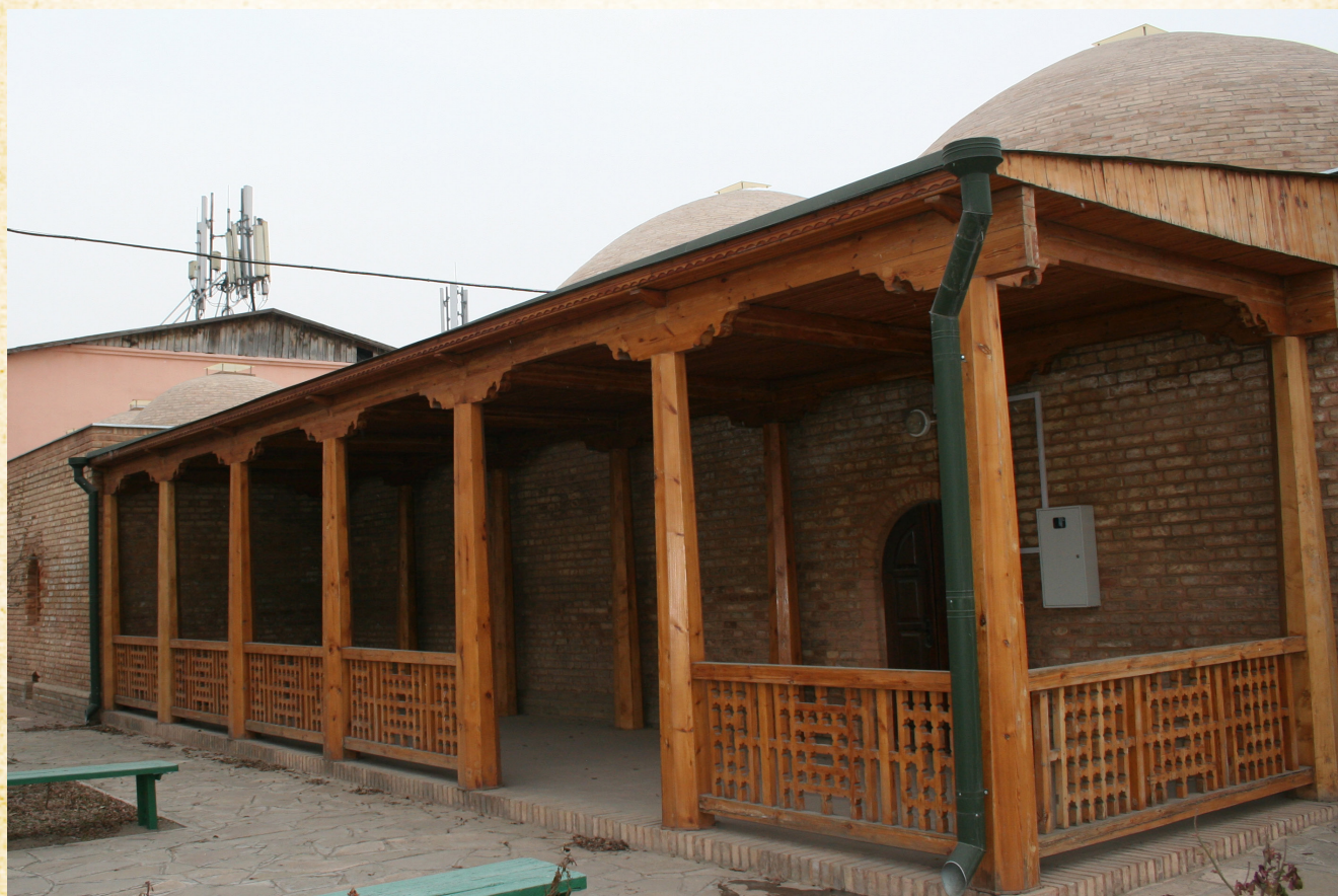
Bath hall of Kali Yunus after restoration, 2016
